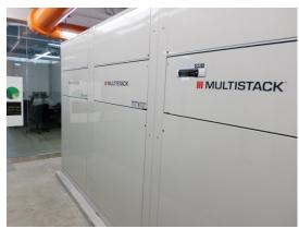
The factory remodel required a more multifaceted approach. Three Multistack dual quad modules (see above) yielding 145 tons, are used for making ice, hot water heat recovery and also comfort cooling.
