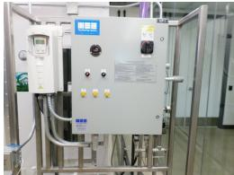
Meefog humidifiers (controls shown above), while used primarily in the Skyline units, are also found in ductwork for the Office spaces. Meefog systems use high-pressure water fogging technology that humidifies and cools the air without need of steam, producing a highly efficient and reliable system.
